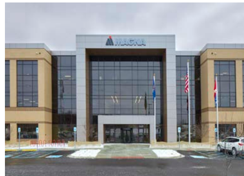
Magna's new seating HQ is a three-story building with 180,000 square feet of space.
